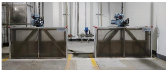
图5 格栅闸门密闭加罩现场 Fig. 5 Site of Airtight Cover for the Grille Gate
